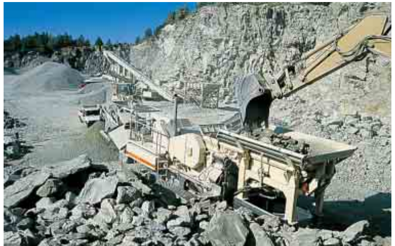
Contract crushing with the Lokotrack LT105S - Norway.
